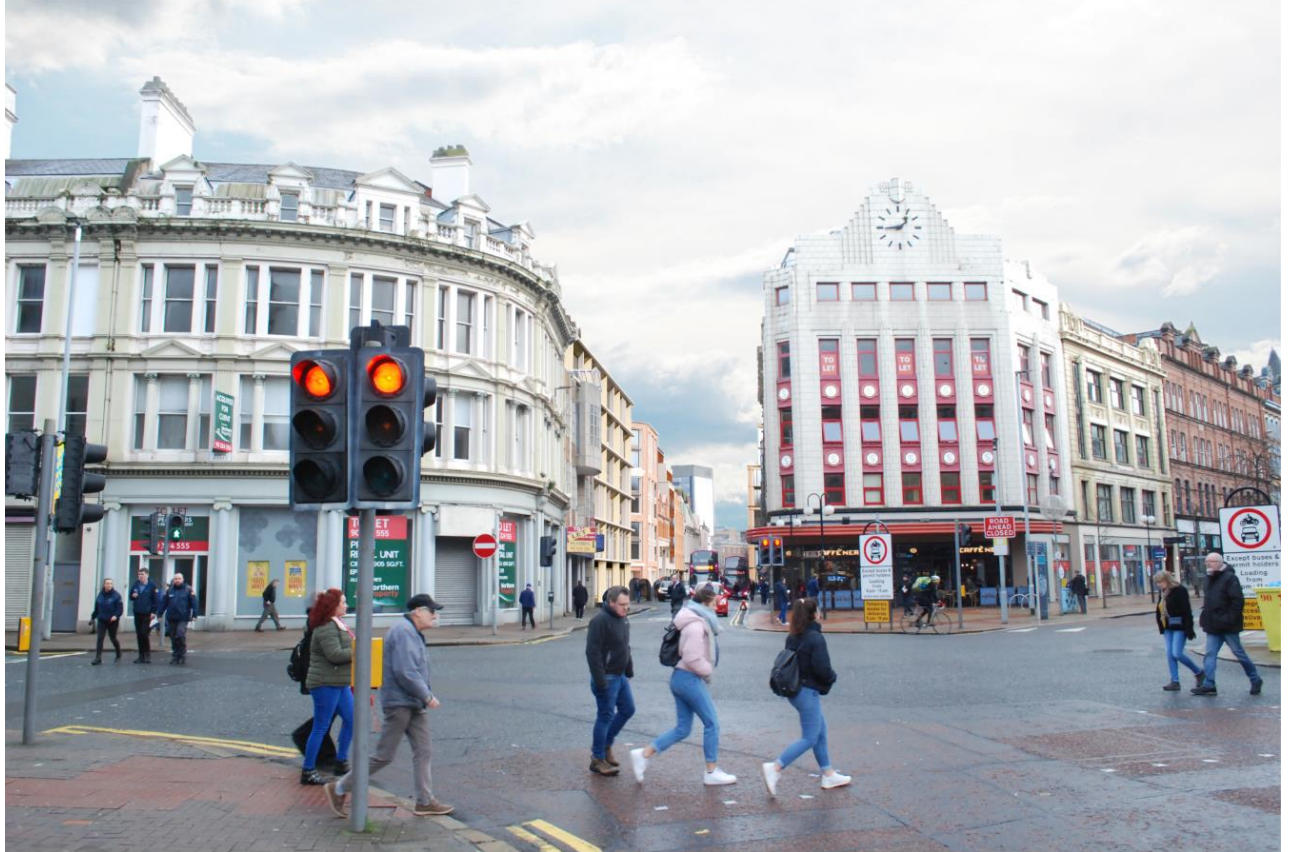
CGI View at the junction of North Street and Royal Avenue
