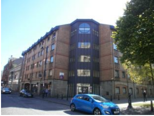
32-40 DONEGALL STREET (SHAC HOUSING)
