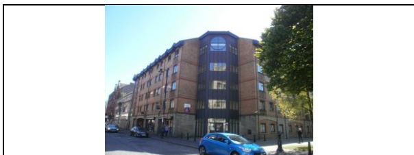
32-40 DONEGALL STREET (SHAC HOUSING)
